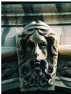
Detail of the facade of the historical Ismailiyya building.
